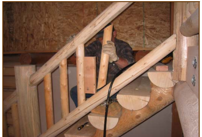
Attach with construction adhesive and nails
