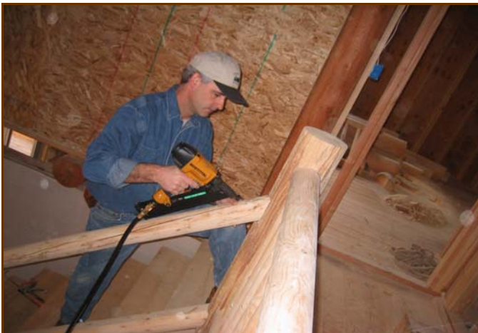
Attach with construction adhesive and nails
