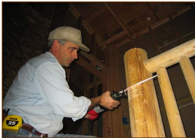
Plunge to notch mark, then remove with chisel
